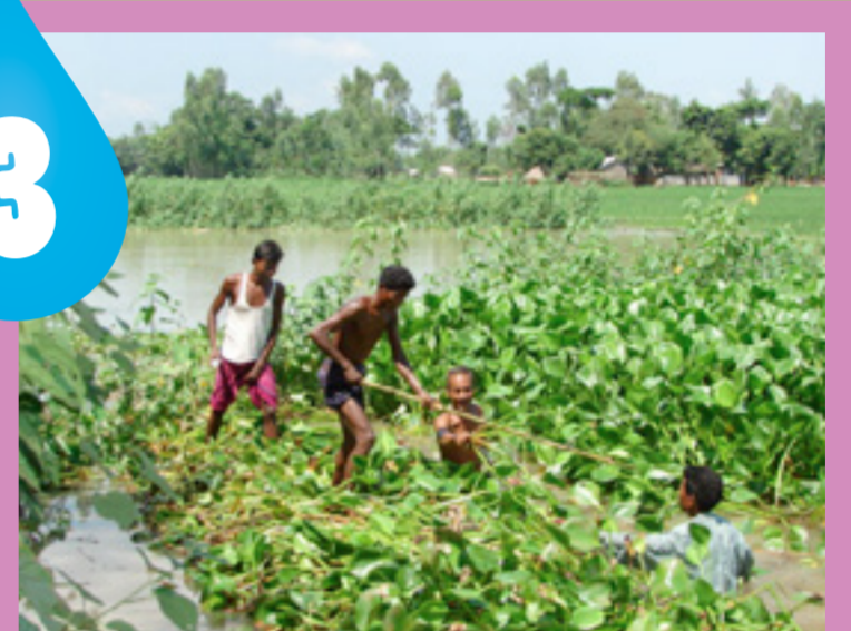
More water hyacinth is woven over the poles to make a basic raft structure of around 8 x 2 metres.
