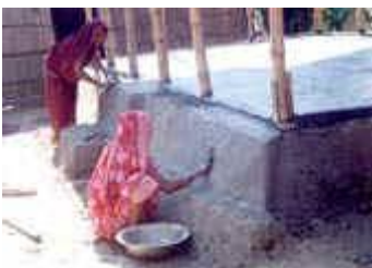
Figure 2: Finishing off the plinth. Photo: Practical Action Bangladesh.
