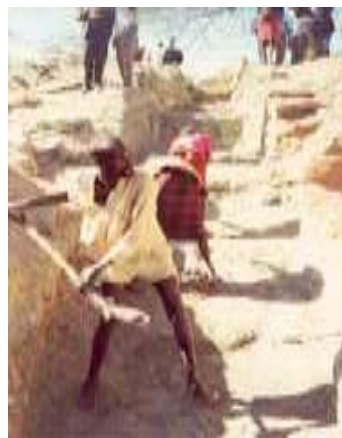
Figure 4: Community involvement in sand dam construction
