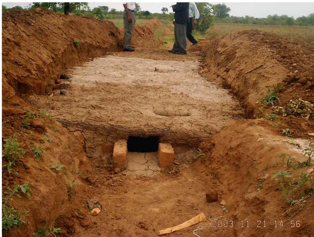
Figure 3: 10 m<sup>3</sup> water storage facilities to avoid evaporation & deep percolation
