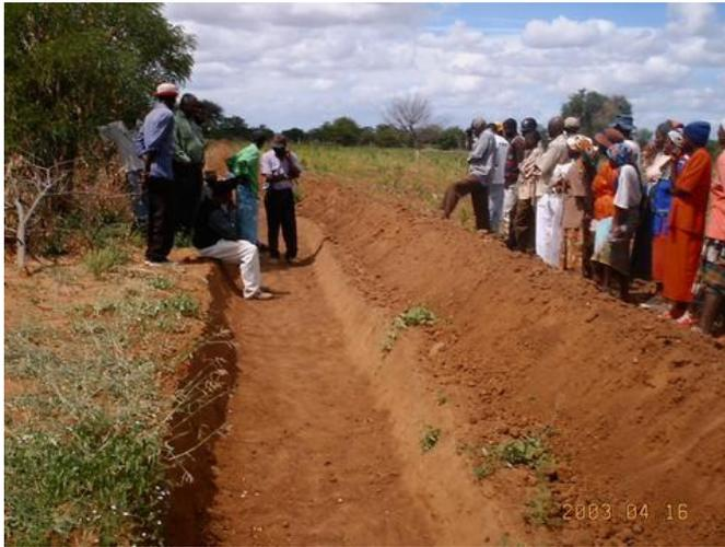
Figure 2: Complete dead level contour ready to harvest water.
